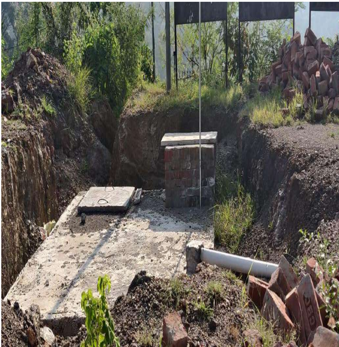
Photograph 12 Rainwater Harvesting Tank with connections for gardening
